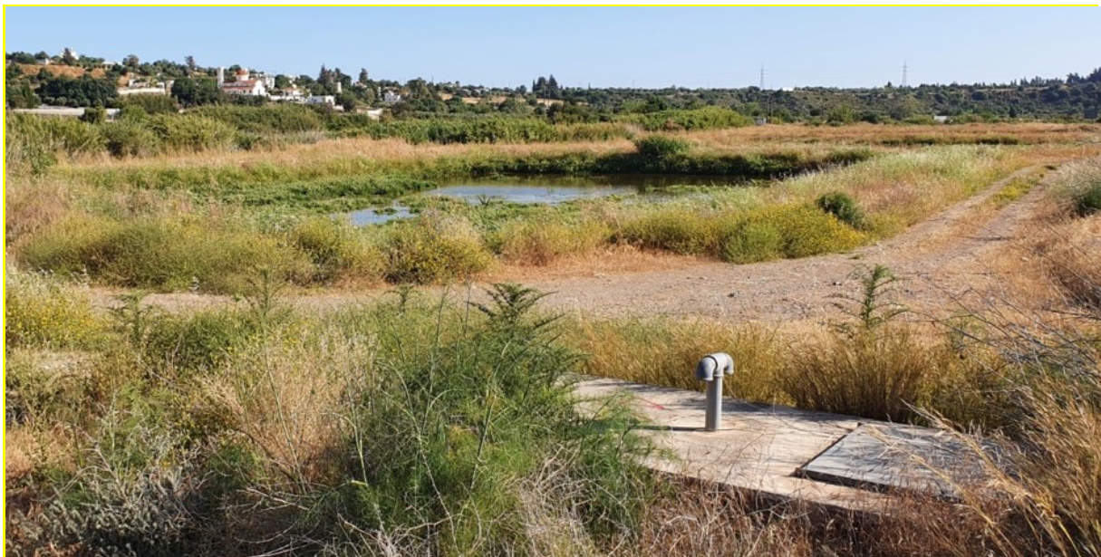
Figure 1. Infiltration pond at Ezousas MAR scheme in Cyprus
